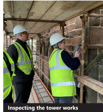
Inspecting the tower works
